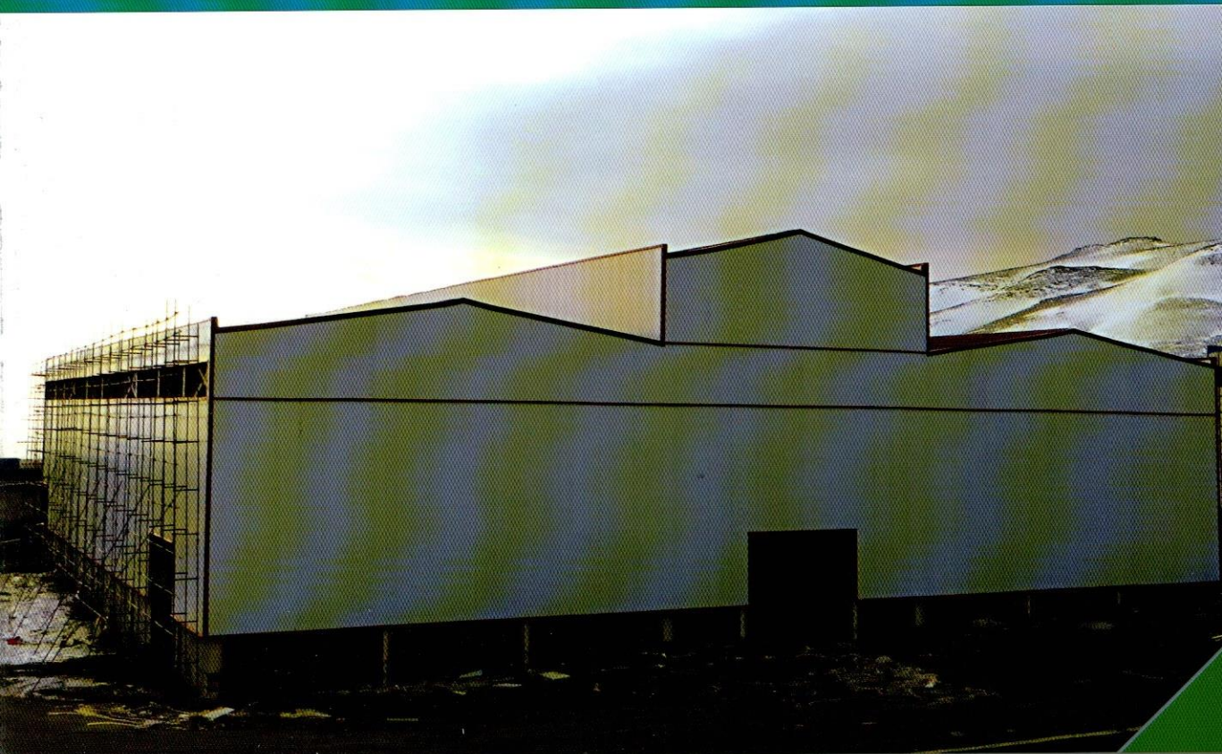
Roof of dairy center in Cremona
